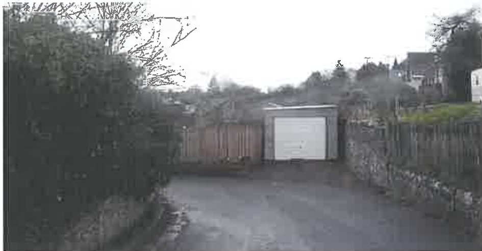
Photo 12 – The Loan at Bend to Left
